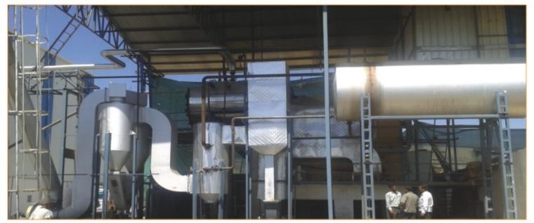
This is a unique design membrane water wall type boiler combining the advantages of water tube & smoke tube designs. Proven technology of fully sealed water wall membrane, which is used worldwide for better heat recovery, has been incorporated to provide high efficiency in this model.
